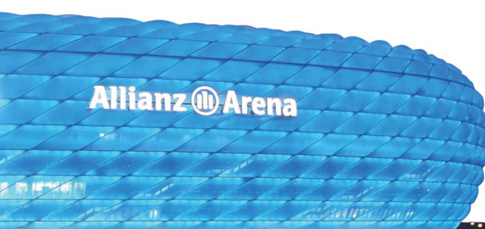
Fluon® ETFE FILM used for the Allianz Arena, a soccer stadium in Germany
