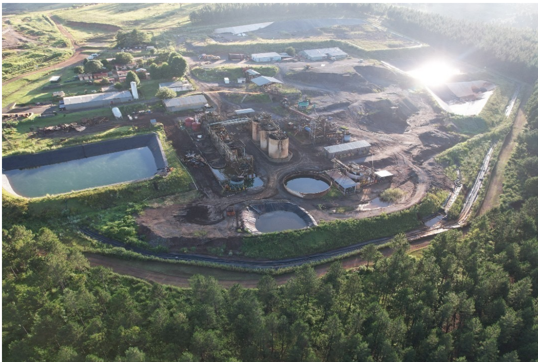
Figure 13: Existing Plant Drone View (post demolition of old sections)
