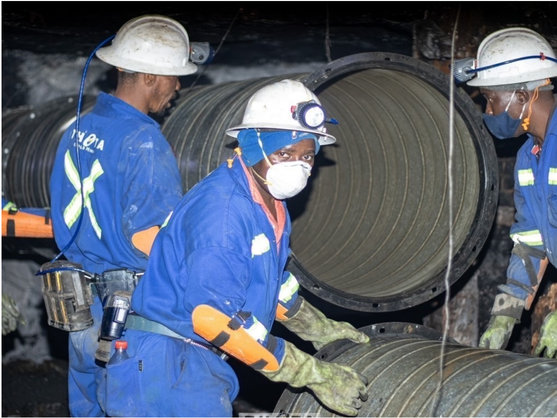
Figure 19: Underground miners installing ventilation piping for Frankfort gold mine
