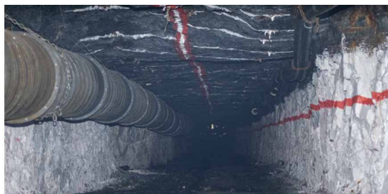
Figure 4 & 5: Miners installing pipe ventilation at Frankfort mine
