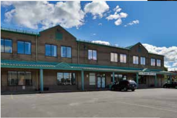
315-325 Macdonald Street, Saint-Jean-sur-Richelieu
