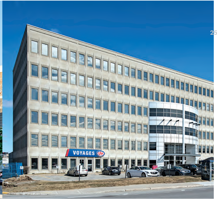
3131 Saint-Martin Blvd West, Laval
