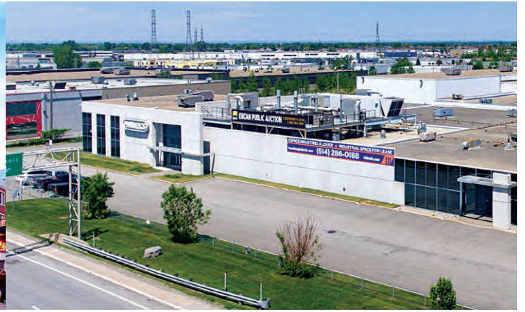
3695 Des Laurentides (Highway-15), Laval
