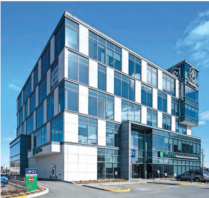
3111 Saint-Martin Blvd West, Laval
