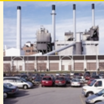
A new enclosed coal-conveyor system at Blount Generating Station improves efficiency and controls dust and sound.
