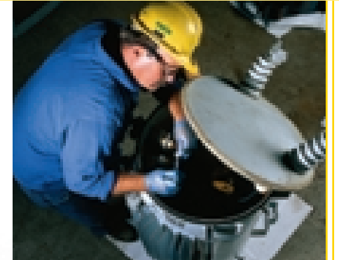
Eliminating PCBs in transformers is one goal of MGE’s new Environmental Management System. MGE Line Technician Steve Anderson tests transformers for PCBs.
