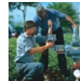
Improved customer service and efficiency are goals of MGE’s automated meter reading (AMR) system. Joe Gary (right), MGE Superintendent – Gas Measurement, inspects an AMR installation by MGE Foreman Mark Cunningham.
