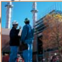
Tim Bliefert (left), MGE Construction Management Engineer, and Rodney Washington, President and CEO of Proactive Safety Consultants, review progress on MGE's West Campus Cogeneration Facility. The plant is on schedule to start serving customers by summer 2005.
