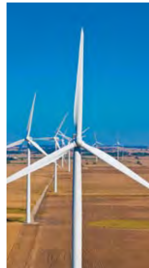
MGE's most recent wind farm has 18 turbines and can produce enough energy to power about 12,000 homes.
