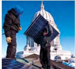
Workers install a set of solar panels on a wing of Wisconsin's state Capitol.
