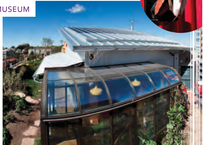
Solar panels provide energy and educational opportunities at the new Madison Children's Museum. A fun feature in the rooftop garden is a chicken that lays eggs based on the amount of solar energy produced.
