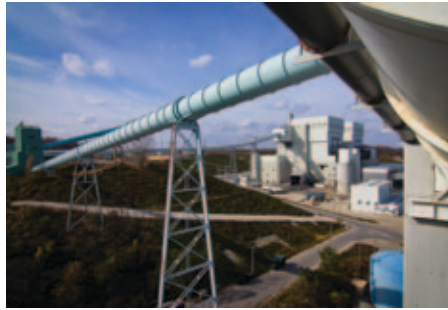
The Elm Road Generating Station's second unit came online in January 2011.
