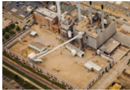
Blount Generating Station's coal yard is now vacant because the Madison plant uses only cleaner-burning natural gas.
