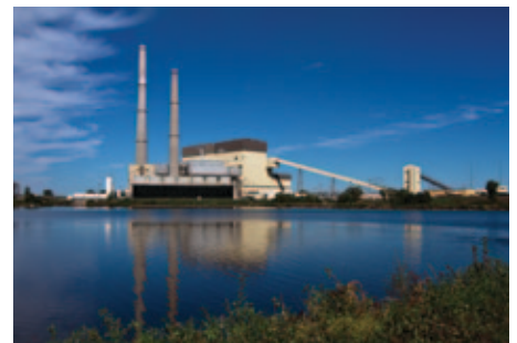
Construction of new emission controls for the Columbia Energy Center will begin this spring.
