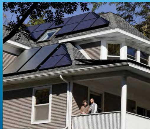
Since 2007, MGE customers Jean and Jonathan Patz have collected solar energy on their roof. Their photovoltaic installation also feeds clean renewable energy to MGE's community energy grid.
