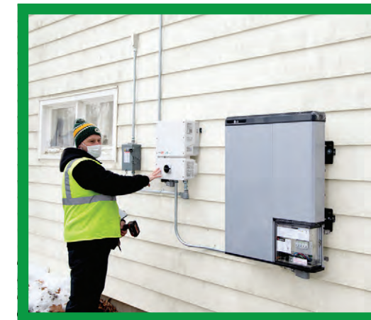
The residential battery, installed on the exterior of the home, is charged by the home's rooftop solar system. The project will help MGE better understand how battery technology could be used to manage peak demand and to enhance reliability.
