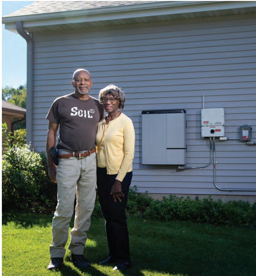
Birl and Ester Lowery, at their home on the west side of Madison, are helping MGE test a residential battery storage unit that is connected to their home's rooftop solar panels and MGE's distribution grid.
