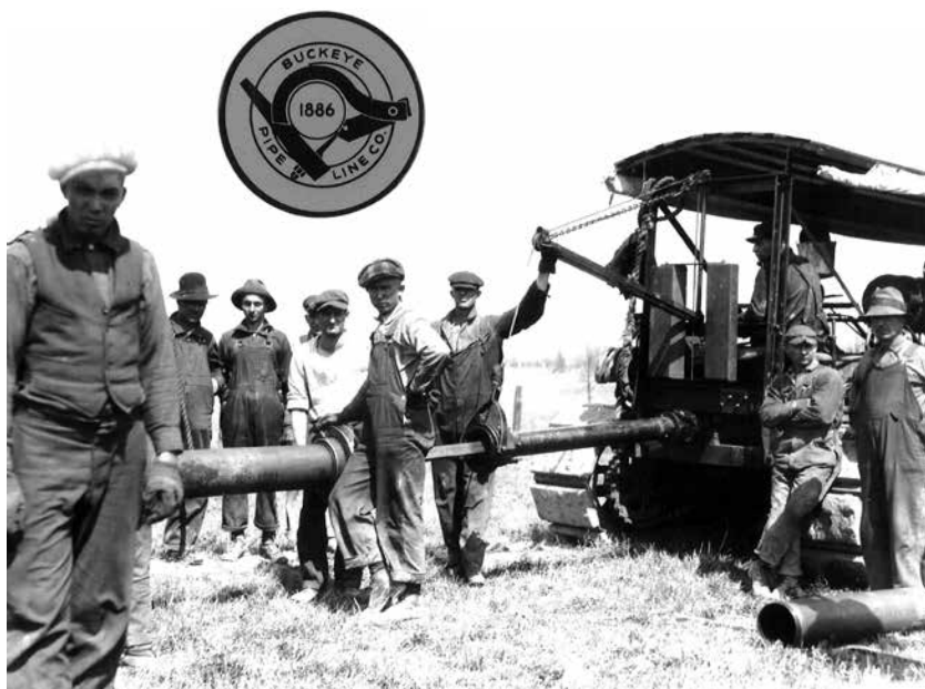
Buckeye construction crew utilizing crawler tractors for pipeline construction in the early 20th century
