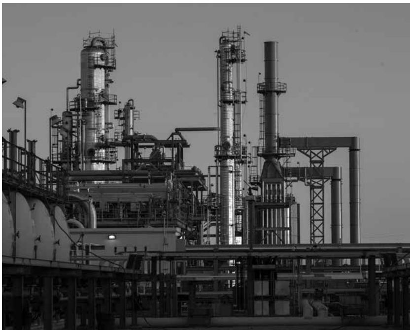
Newly commissioned condensate splitter at Buckeye Texas Partners' facility
