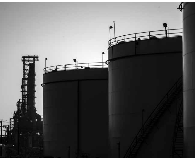
Crude and kerosene product storage tanks at Buckeye Texas Partners' facility
