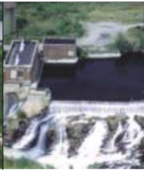
Riverside Dam New Hampshire
