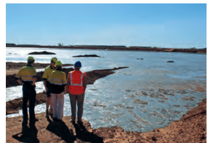
Inspection of new tailings storage facility at Ellendale
