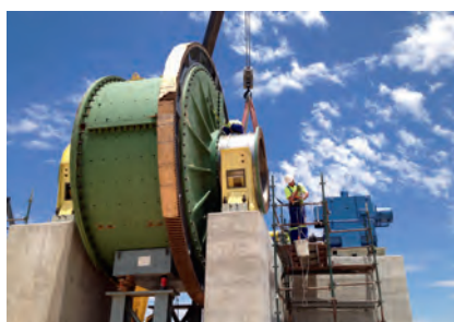
Installation of the autogenous mill at Ghaghoo
