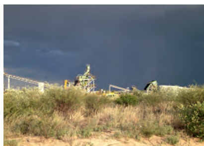
Treatment plant at Ghaghoo
