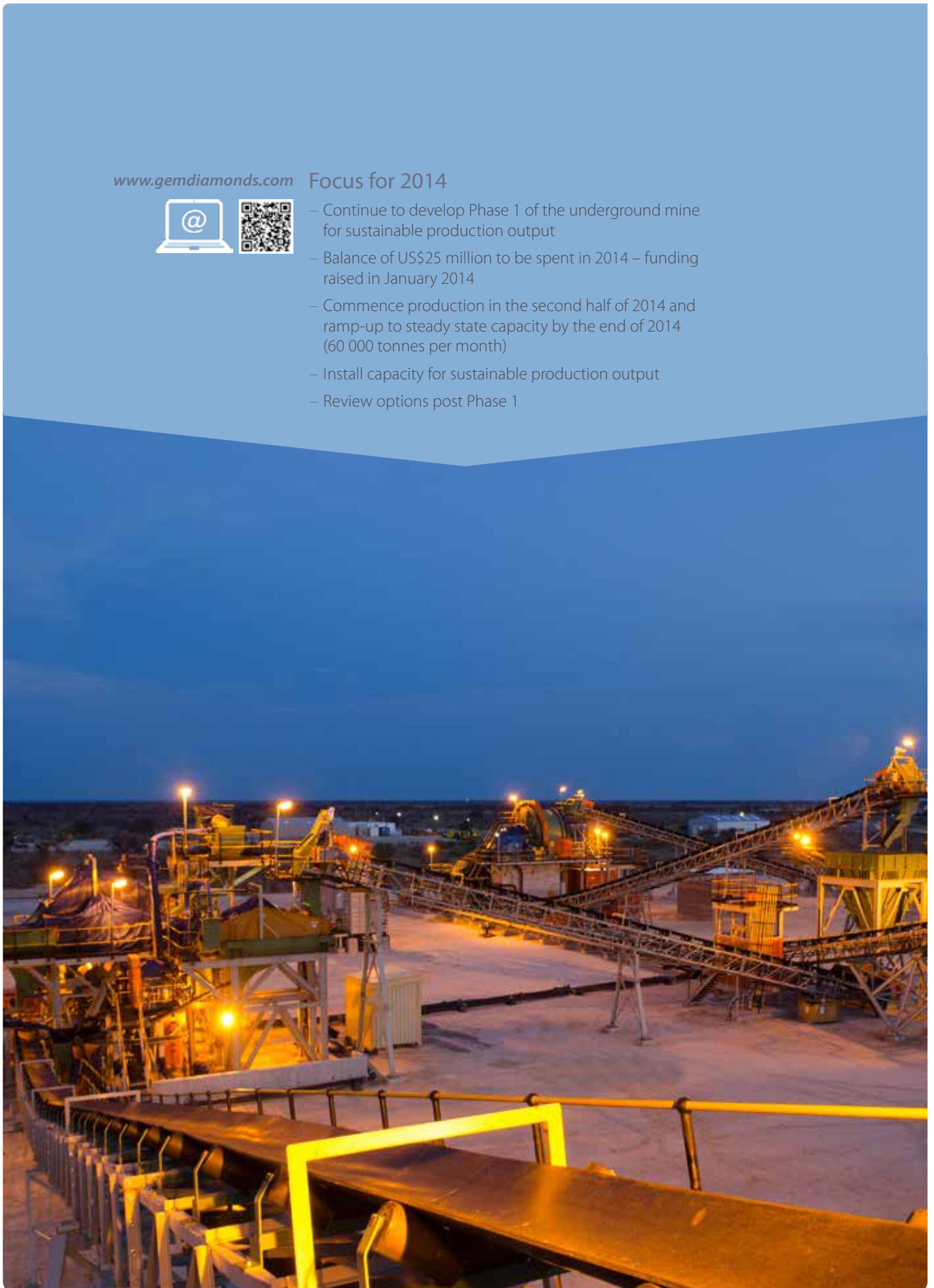
The processing plant at Ghaghoo is complete and ready for final commissioning.
