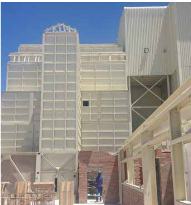
Construction of the new Coarse Recovery Plant under way.
