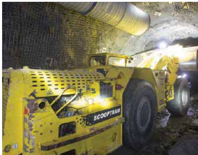
Underground equipment in the kimberlite tunnels in level 1.
