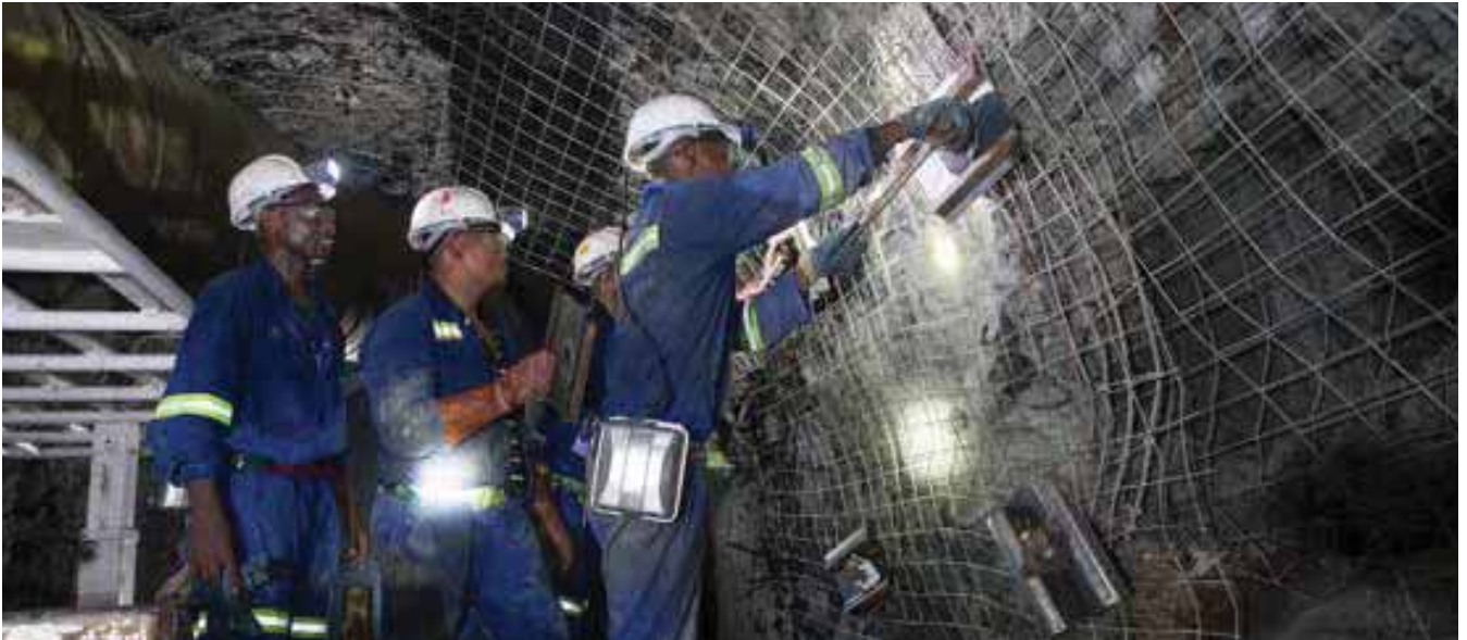
Lining the kimberlite tunnels with safety meshing.
