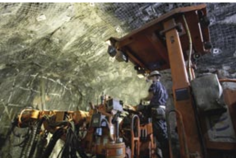
Single-person operated Jumbo at Marvel Loch Underground
