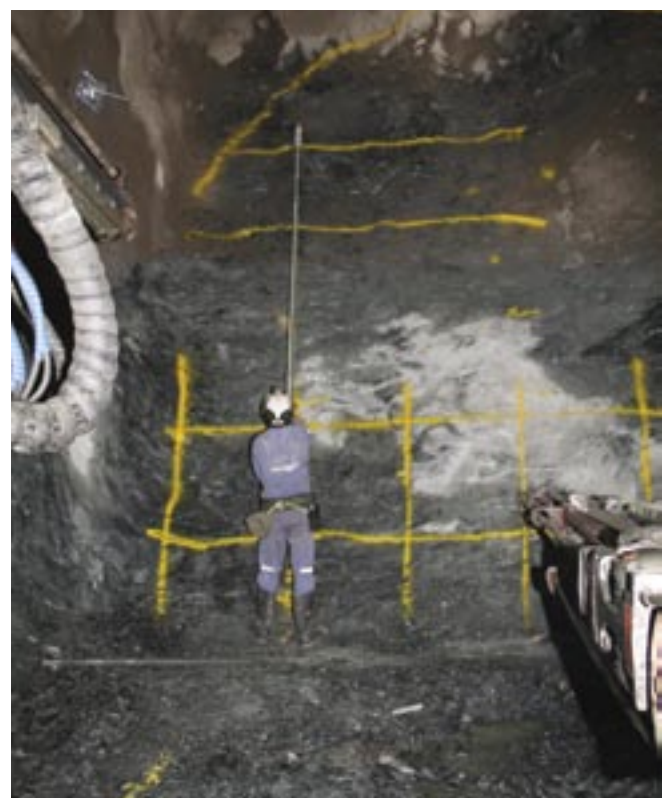
Preparing the face for next advance of Hoover Decline, 5.8m high by 6.0m wide
