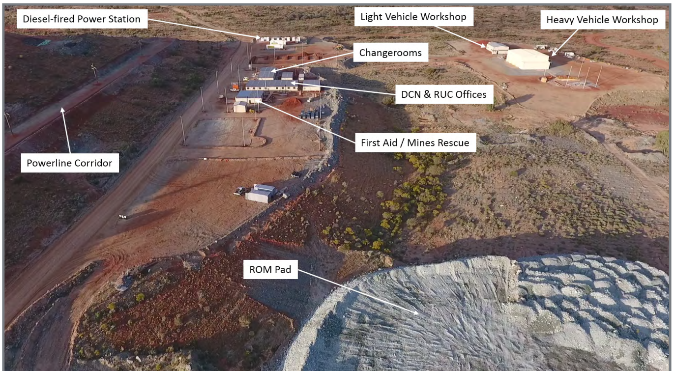
Figure 6: Aerial view of the Westralia Mine Service Area layout and construction. Key sections are labelled.
