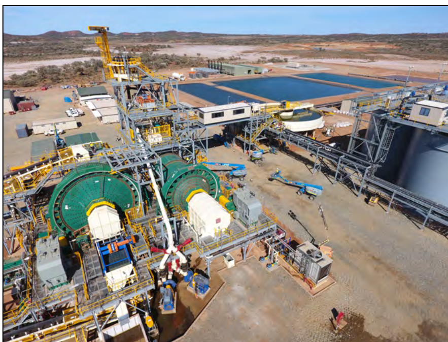
Figure 4 SAG mill and ball mill assembly with CIL tanks of the new 2.5Mtpa treatment plant at MMGO. Note the treatment plant ponds and power station behind the mills and tanks.
