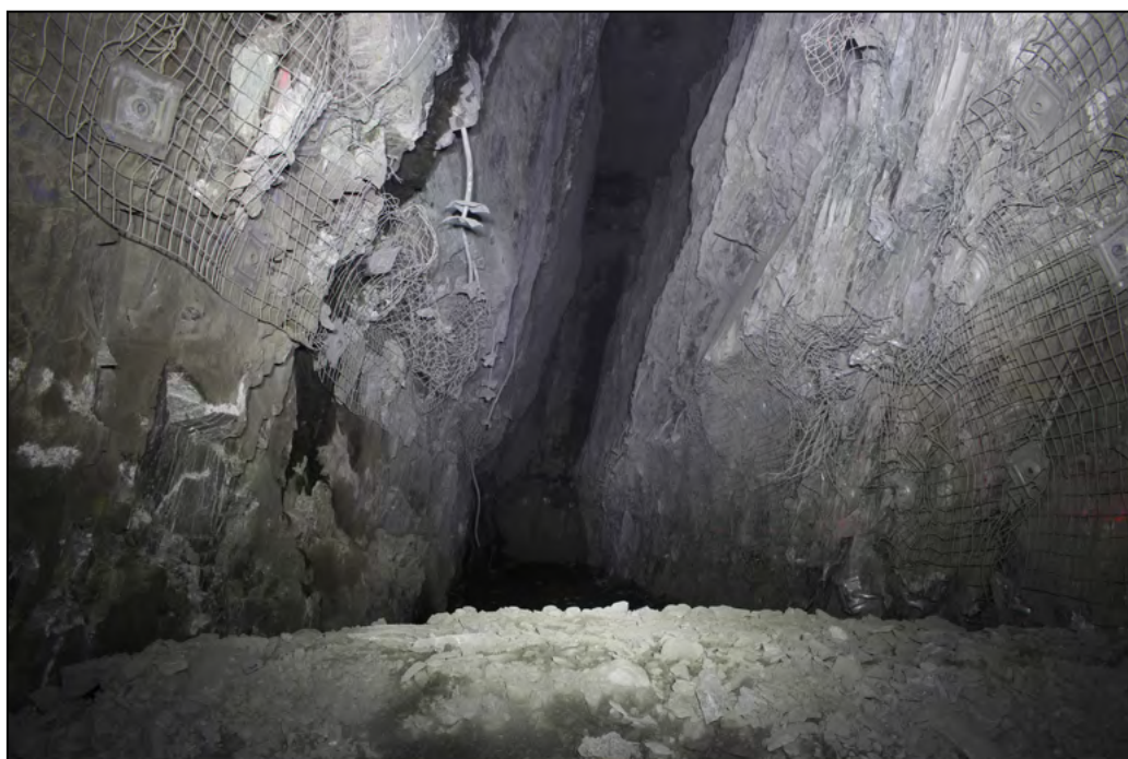
Figure 7 Good stopping conditions at Beresford South
