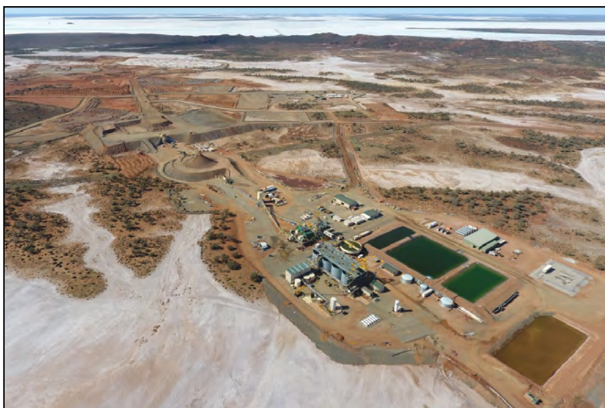
Figure 3 Aerial view of the 2.5Mtpa treatment facility at MMGO
