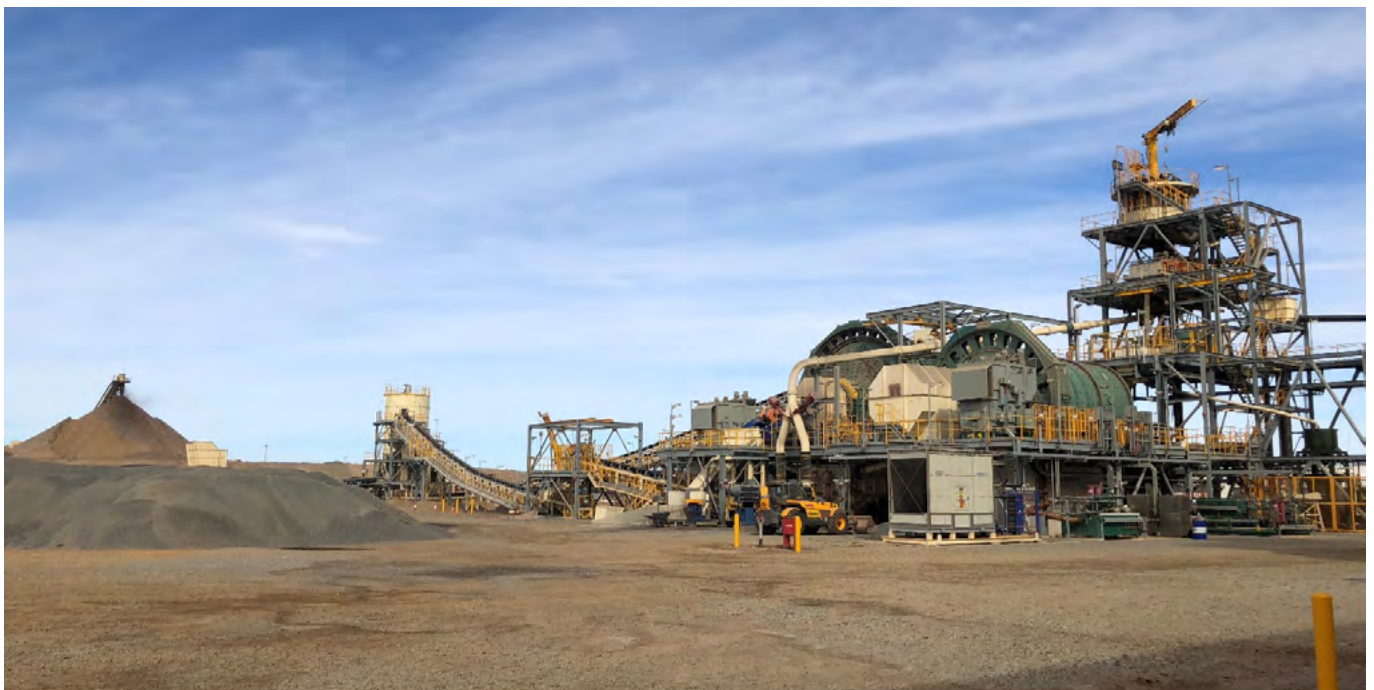
Figure 5: Coarse ore stockpile, SAG and ball mill assembly
