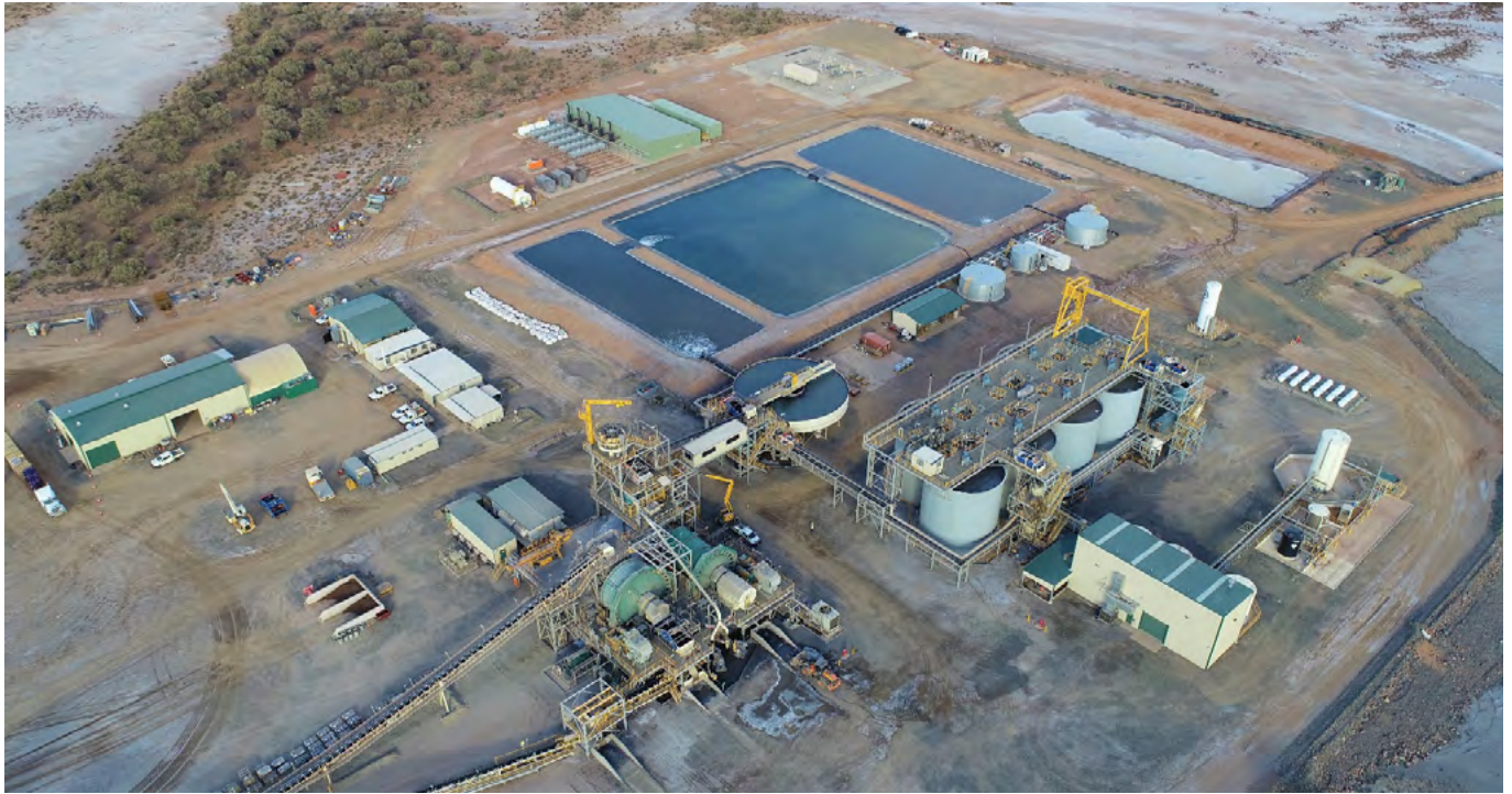
Figure 4: Aerial view of the back-end of the 2.5Mtpa treatment plant at MMGO showing ball and SAG mills; CIL tanks, gold room, water storage and the gas-fired power station
