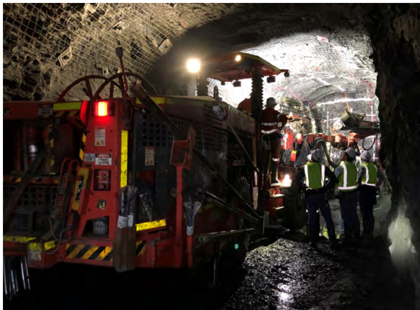
Figure 7: Underground jumbo development
