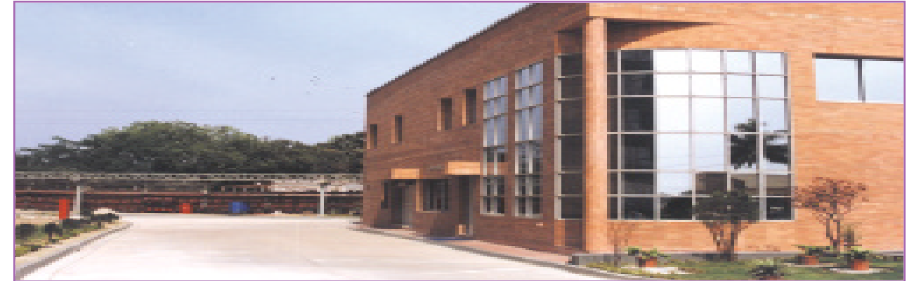
State-of-the-Art MDI Plant, Tongi, Gazipur
