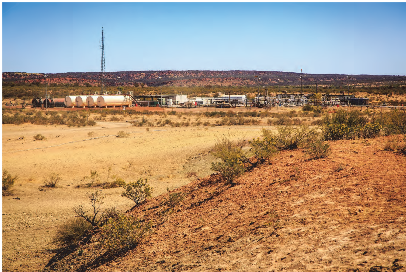
Mereenie Eastern Satellite Station Processing Facilities
