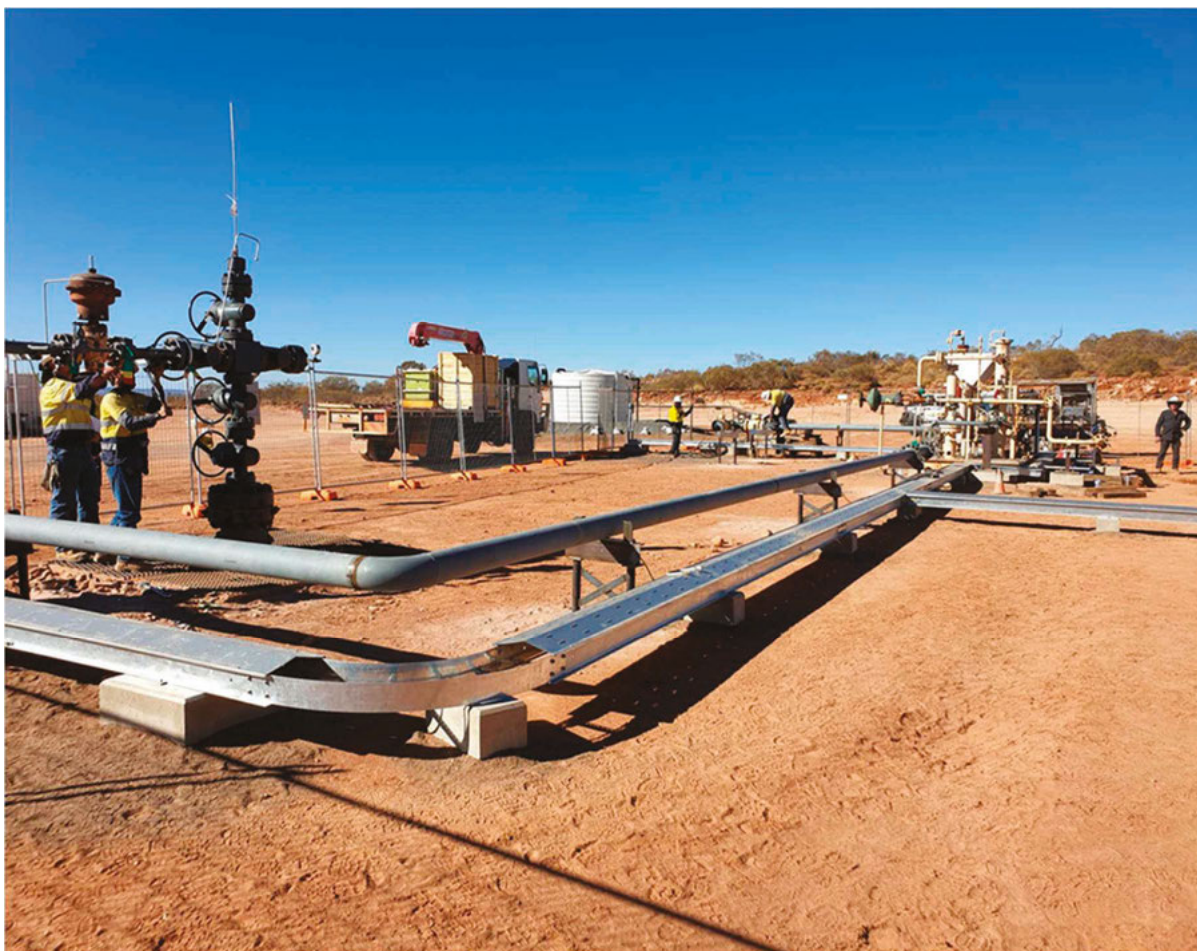
Palm Valley-13 well during commissioning
