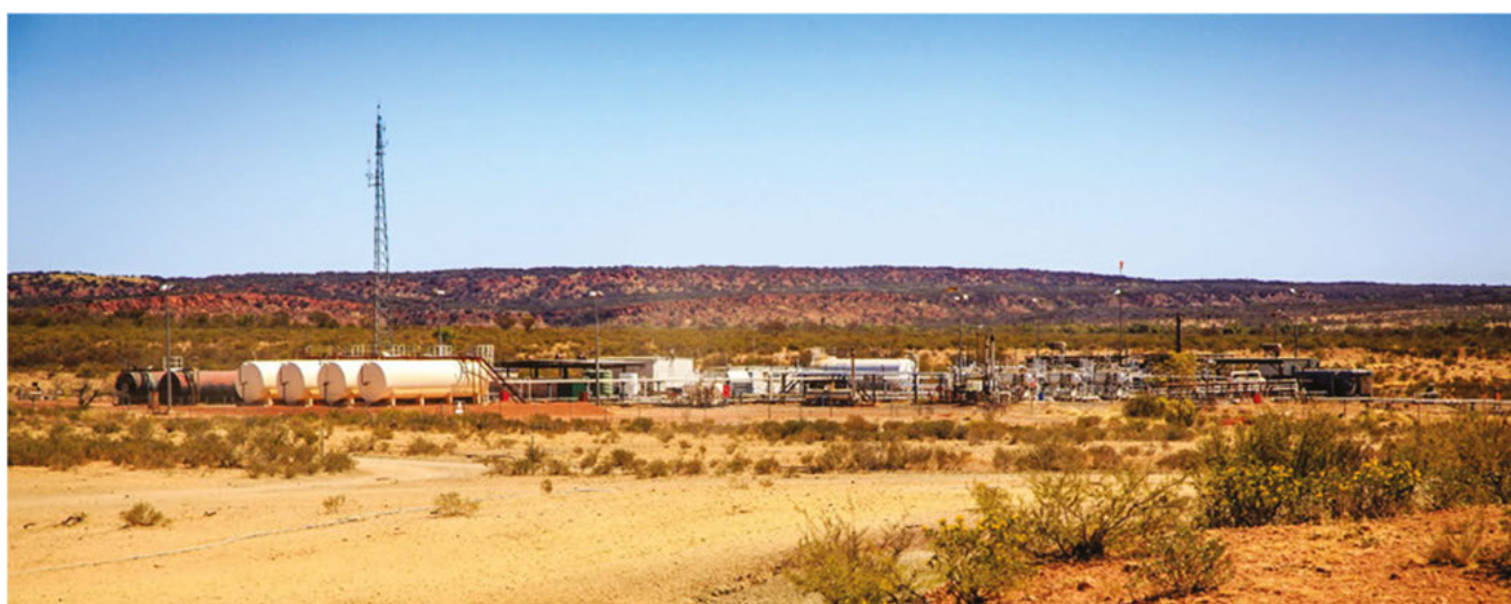
Mereenie Eastern Satellite Station Processing Facilities
