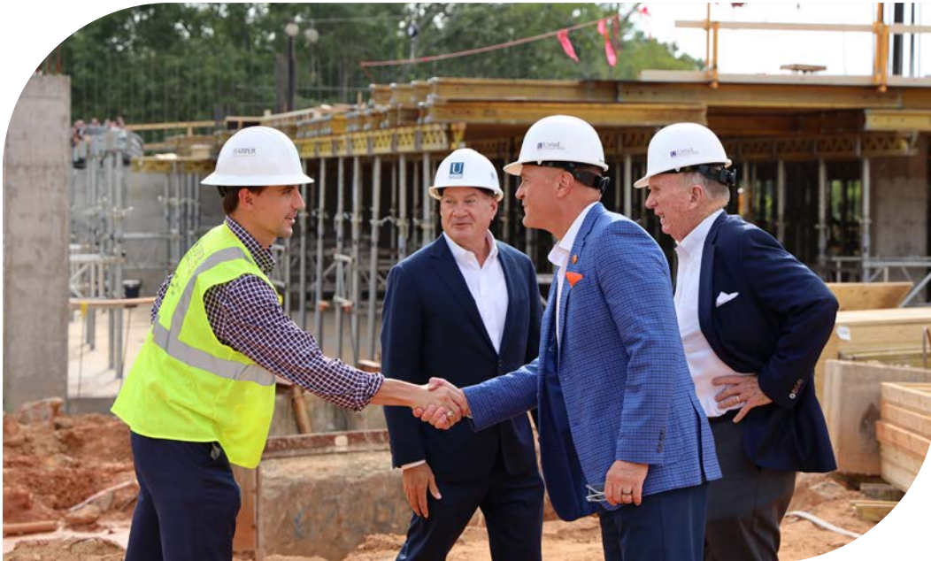
The board visits the construction site of United's new headquarters in Greenville, SC.
