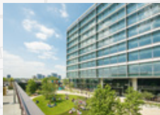
Paddington Central 11 acre office-led campus close to Paddington Station
