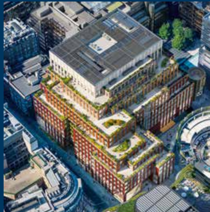
▲ 1 Broadgate Office-led redevelopment at Broadgate including 46,000 sq ft of retail connecting Finsbury Avenue Square with 100 Liverpool Street and the Broadgate Circle to create a retail, leisure and dining hub. Office space is fully pre-let or under option to JLL and Allen & Overy.
