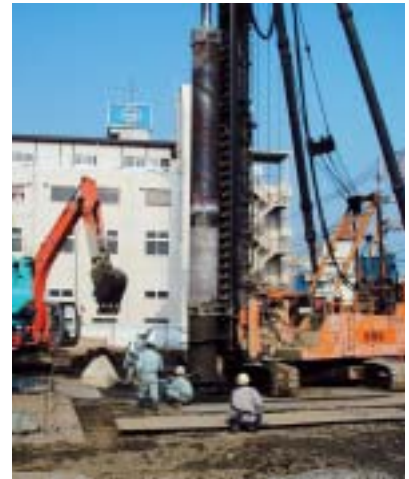
DynaWing™ installation
