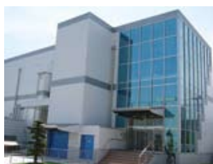
Pellicle plant in Nobeoka
