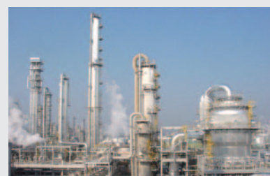
AN plant in Korea
