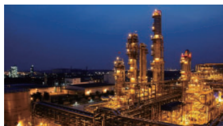
AN plant in Thailand
