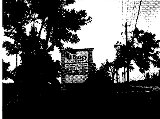
Busey Bank on Summerlin Lakes Dr. in Ft. Myers received damage to signage and landscaping from Hurricane Charley in August. Fortunately, the devastating storms that ravaged Florida during the summer of 2004 did not harm any Busey associates or their families.
