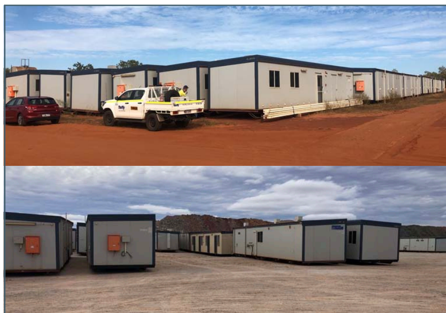
Second-hand portable accommodation units comprising 240 rooms.
