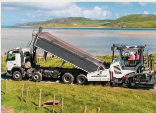
Above: Whitemountain at work on the non-national roads network in Donegal
