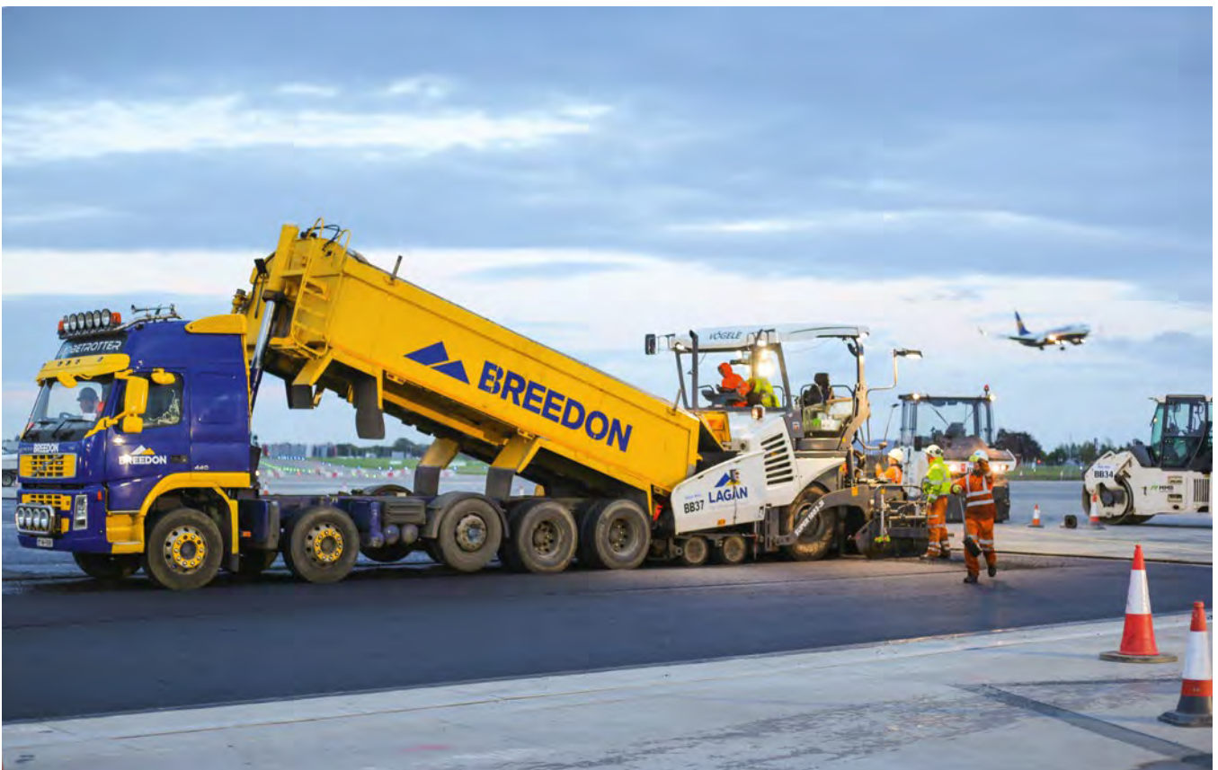
▲ Dublin Airport runway resurfacing project
