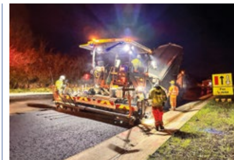
Breedon Group colleagues working on the A11 National Highways contract
