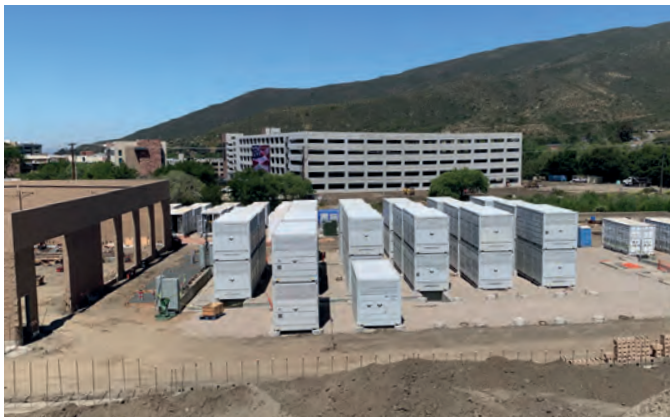
Invinity’s 10 MWh VFB at the Viejas Casino & Resort, the largest VFB in the U.S. – May 2024
