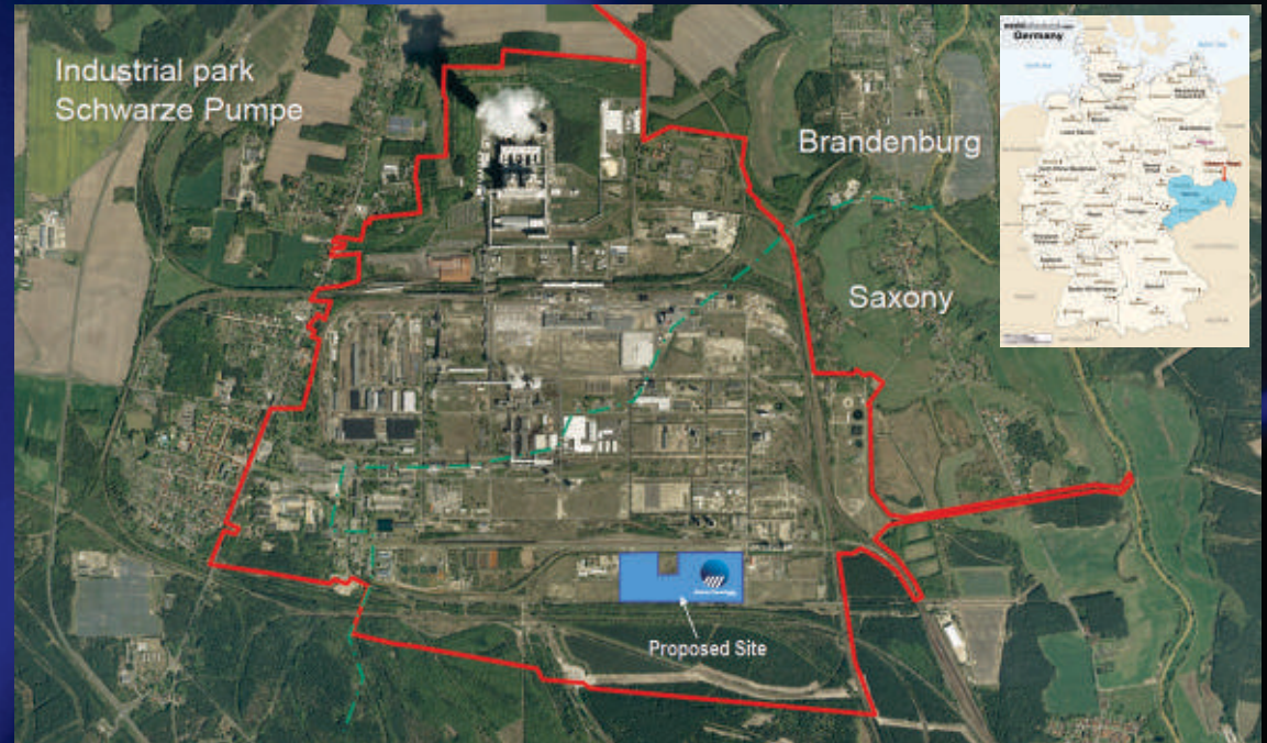
SCHWARZE PUMPE INDUSTRIAL PARK AND THE ~10HA INDUSTRIAL SITE AVAILABLE TO ALTECH
