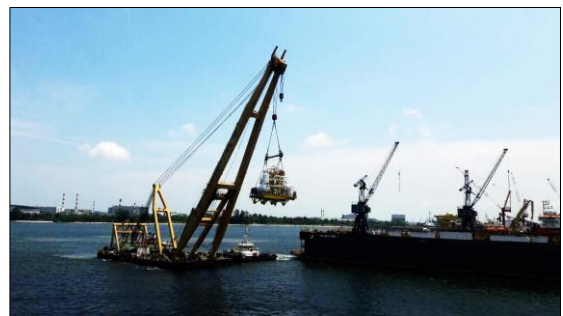
Crude Stabilisation Unit being lifted onto MTC Ledang
