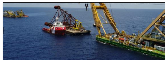
Ophir Platform Installation – Jacket on barge, topsides in background
