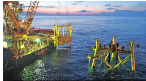
Ophir Platform Installation - Jacket installed, boat landing installation in process
