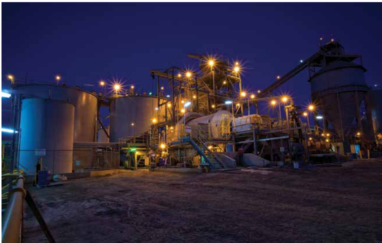
Randalls Gold Processing Facility
