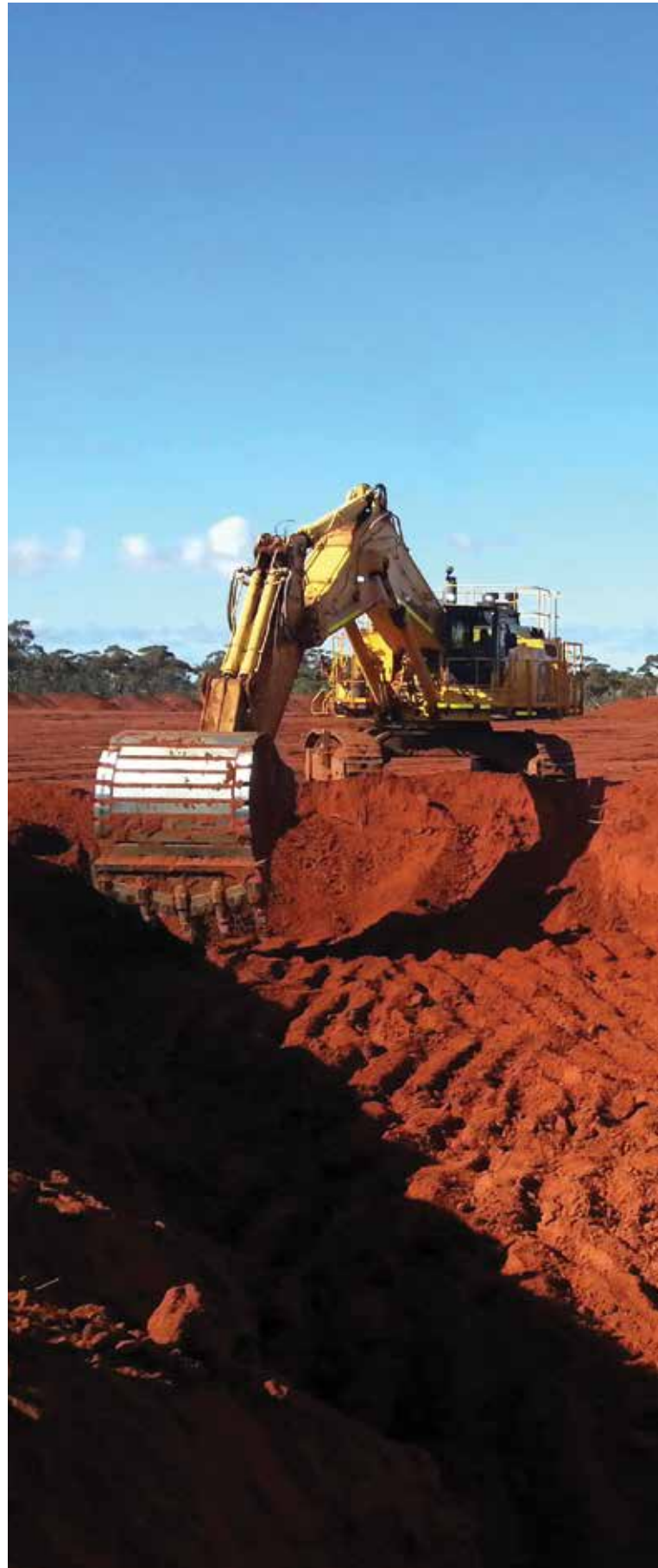
Commencement of Lucky Bay Open Pit
