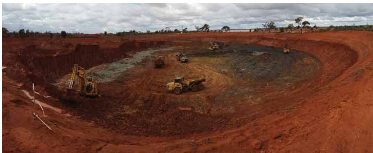
Commencement of Lucky Bay Open Pit
