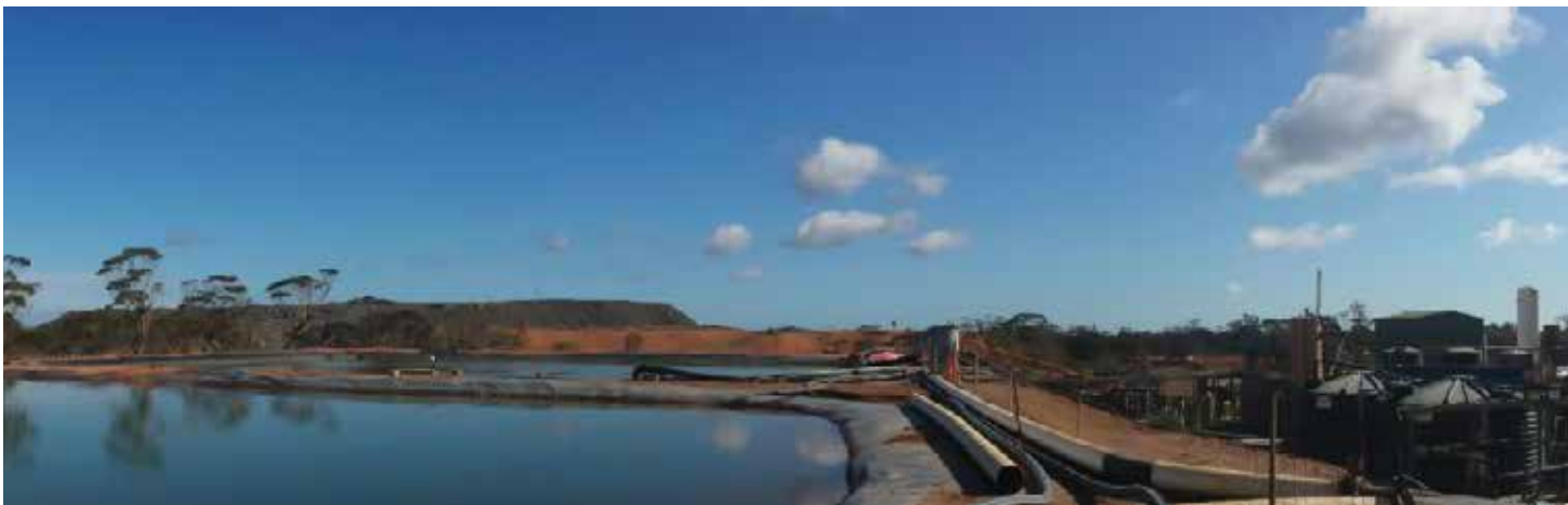
Randalls Gold Processing Facility
