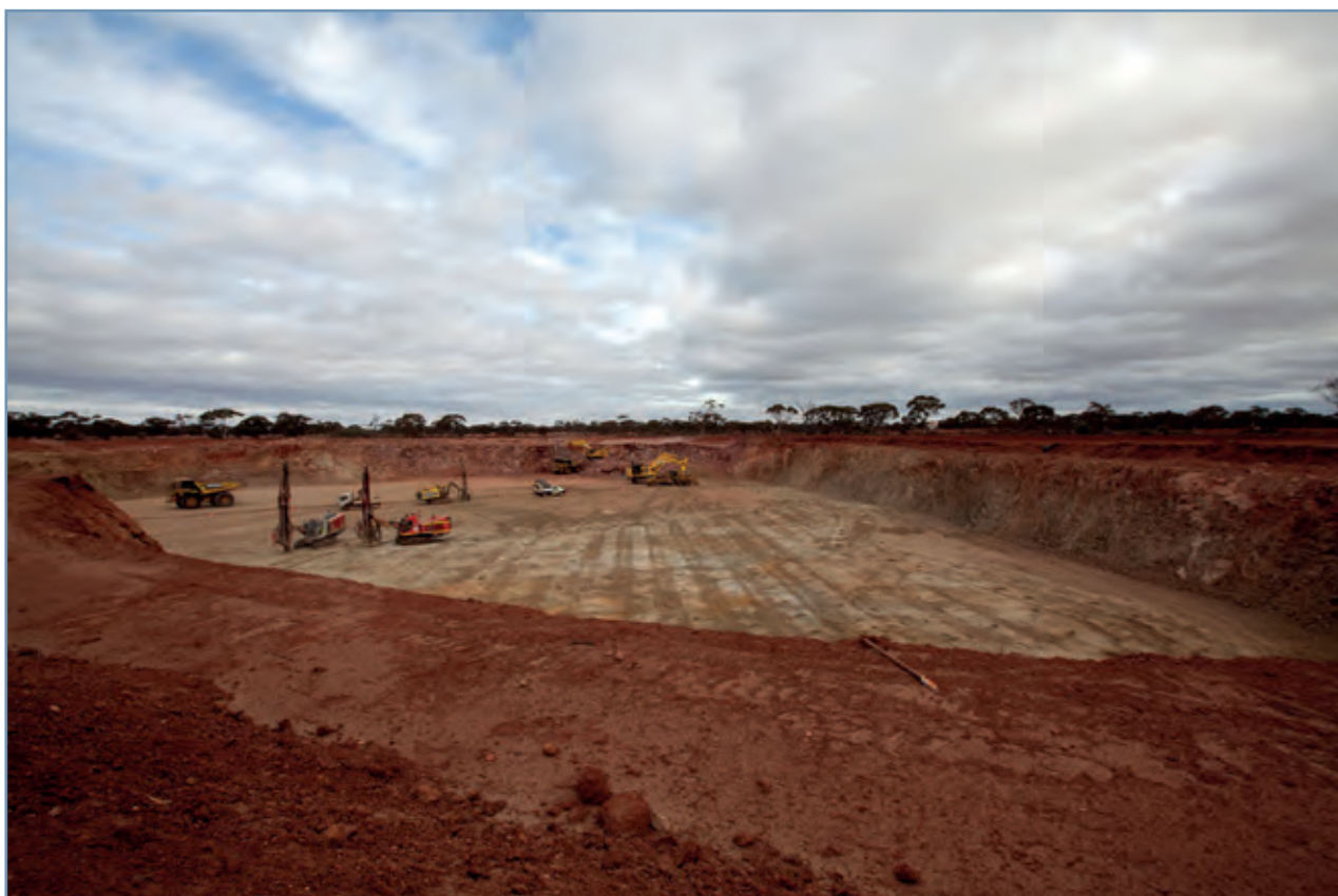
Commencement of Majestic Open Pit
