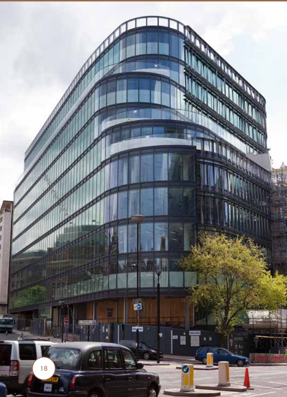
Pictured: 60 Holborn Viaduct
