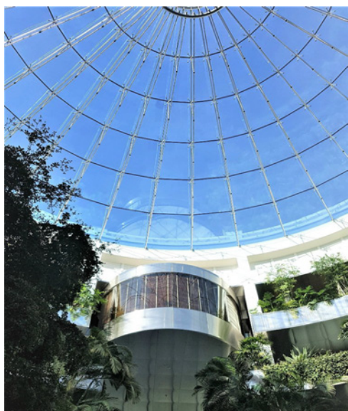
Pereda building. Global Headquarters in Boadilla del Monte (Madrid)
