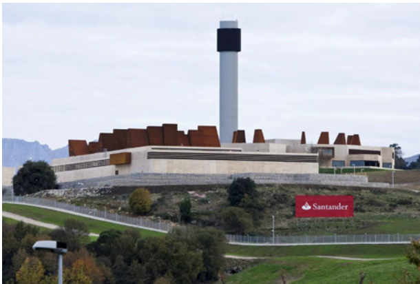
Data centre Cantabria
