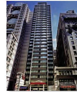
COURTYARD MANHATTAN FIFTH AVENUE
