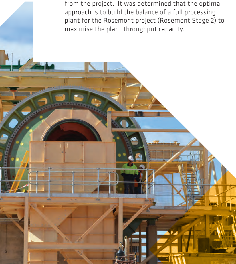
ROSEMONT MILL UNDER CONSTRUCTION
