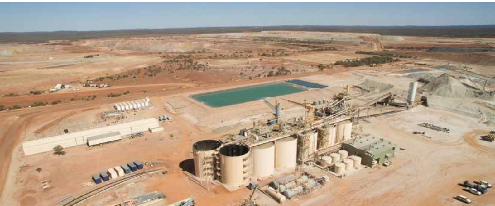
GARDEN WELL PROCESSING FACILITY WITH TWO ADDITIONAL TANKS UNDER CONSTRUCTION
