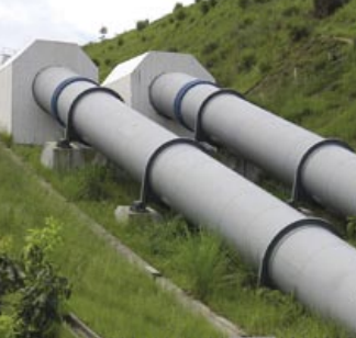
Water Infrastructure Projects in China
